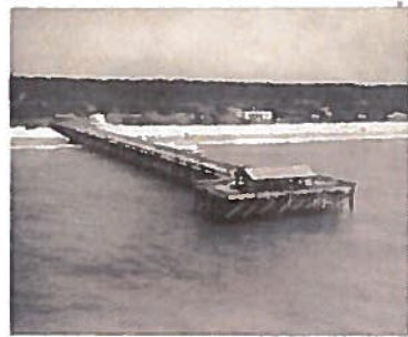
A second chance at new life for the Springmaid Pier in Myrtle Beach, SC. This was how she looked in 1953 when first erected. Look below for the newly rebuilt pier.
