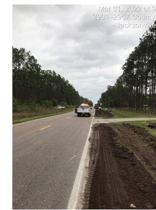
Shoulder repairs on County Road 121
