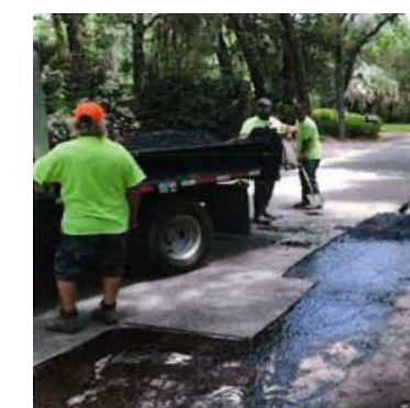
Repairing potholes on Gerbing Road
