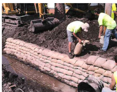
Installing headwall on Nottingham Drive
