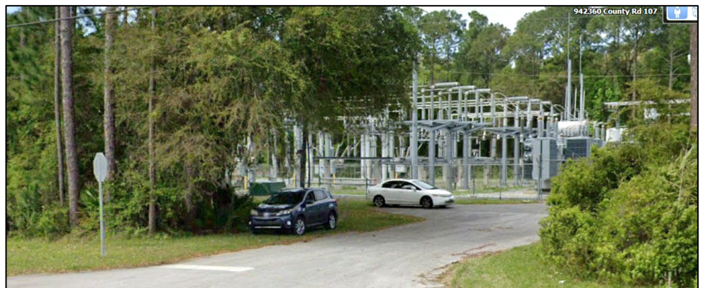
Figure 7: 4.5-acre utility complex located southwest of the subject property
