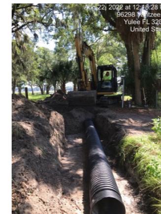
Drainage repairs on Yahtzee Lane
