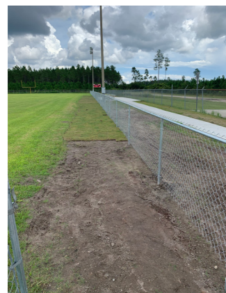
Fence relocation and new sod at Hilliard Ballpark
