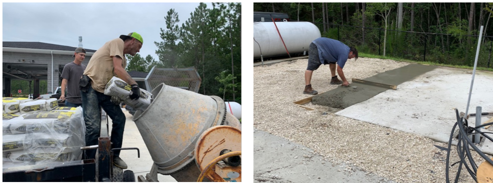
Intalling new concrete pad for new fire station generator
