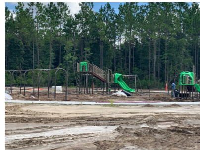
Playground installation at Tributary Park
