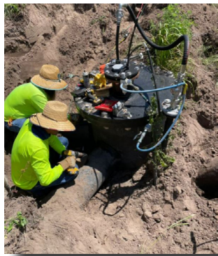
Gas Well Line Repairs
