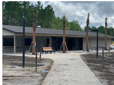
Restroom/concession building installed at Tributary Park, along with new trees, benches and lighting
