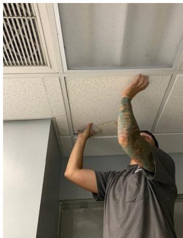
Replacing ceiling tiles at Animal Control
