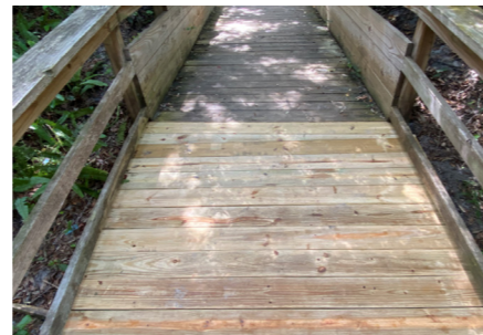
Beach Walkover Repairs
