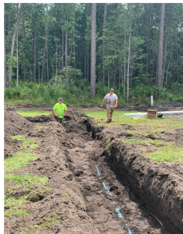
Installing sewer lines
