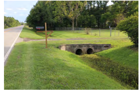
Figure 16: Side Drain Hazard in Clear Zone
