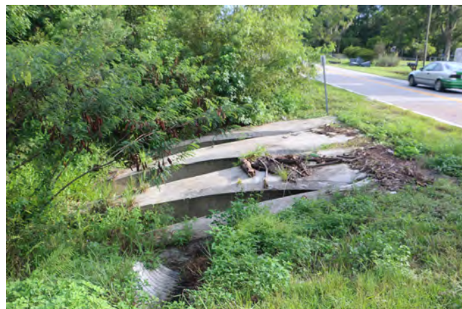
Figure 11: Existing Cross Drain Mitered End Section Within Clear Zone
