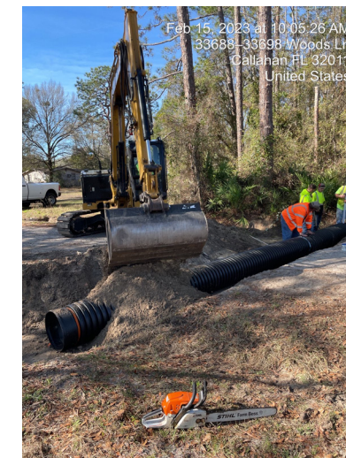
Placing new cross drain on Woods Lane
