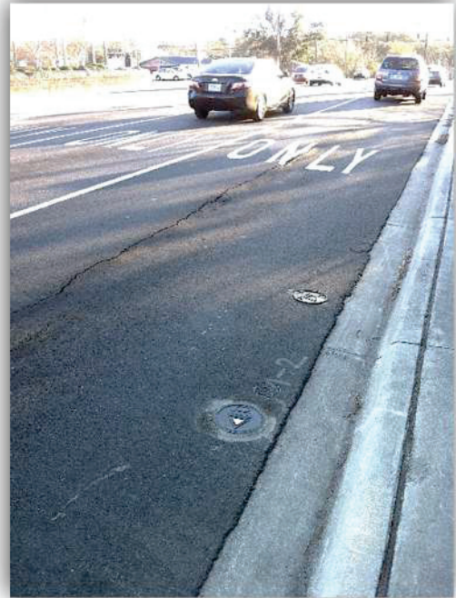
Slope Inclinometers in Roadway
