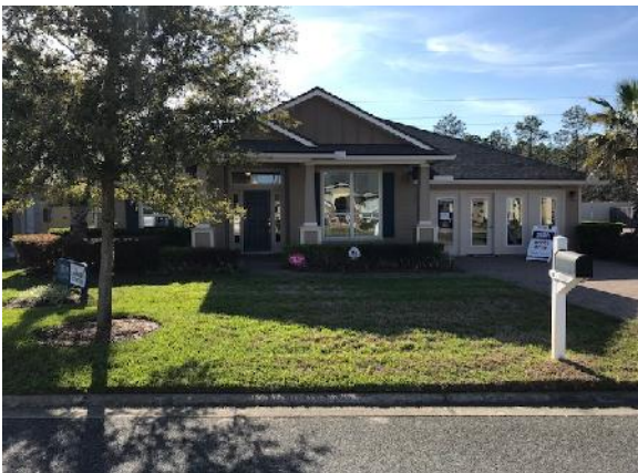
SEDA model home in existing portion of Hideaway (Photo Taken on March 9, 2018)
