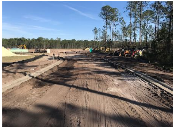
Ongoing Phase 1B development (Photo Taken on March 9, 2018)
