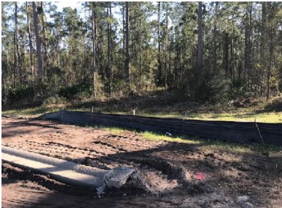
View of Phase 1C from 1B (Photo Taken on March 9, 2018)
